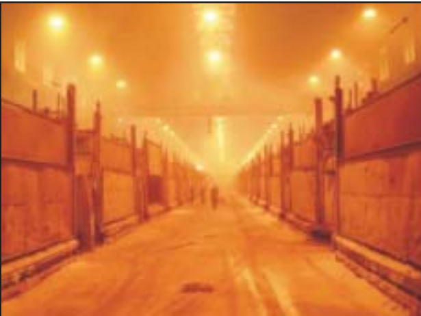
HSS Pot Line at Hirakud Smelter, Hindalco
