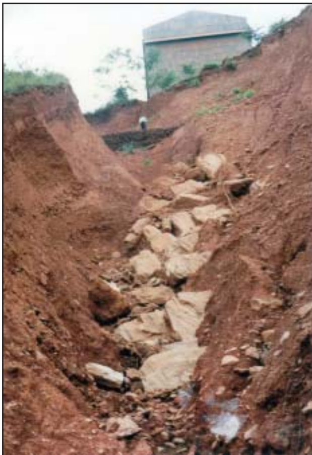
Bund to Arrest Soil Erosion, NALCO
