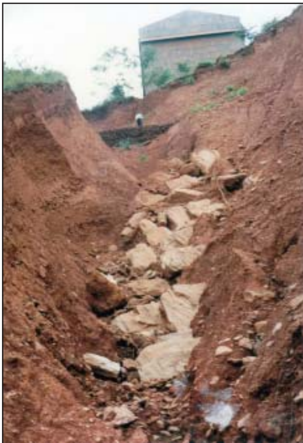
Bund to Arrest Soil Erosion, NALCO
